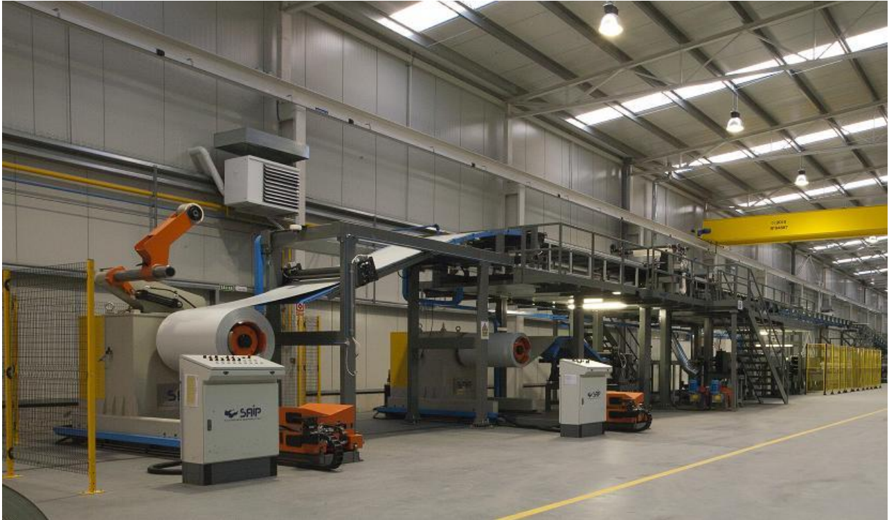
The ce|de|pa continuous production line: the roll forming section.
